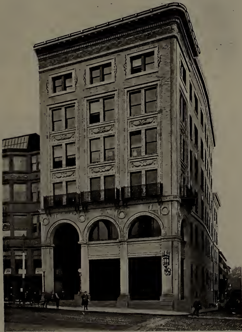
STEINERT HALL BUILDING, 162 to 168 Boylston Street, corner of Carver.
